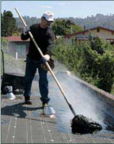
Figure 10. Hot asphalt is mopped onto the base sheet and felt in preparation for the next layer of material (left). These roofers are applying the first full-width piece of felt. There's already a 12-inch and a 24-inch strip below (right).
