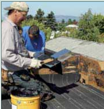
Figure 4. A roofer beds a scupper flashing in roofing cement (left) before fastening it over the base sheet (right).
