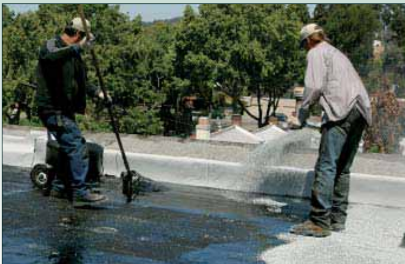
Figure 16. Here, one roofer lays down a thick flood coat of hot asphalt while another spreads crushed granite aggregate on top (left). Since the aggregate protects the roof from UV rays, no asphalt should be visible when the roof is done (above).
