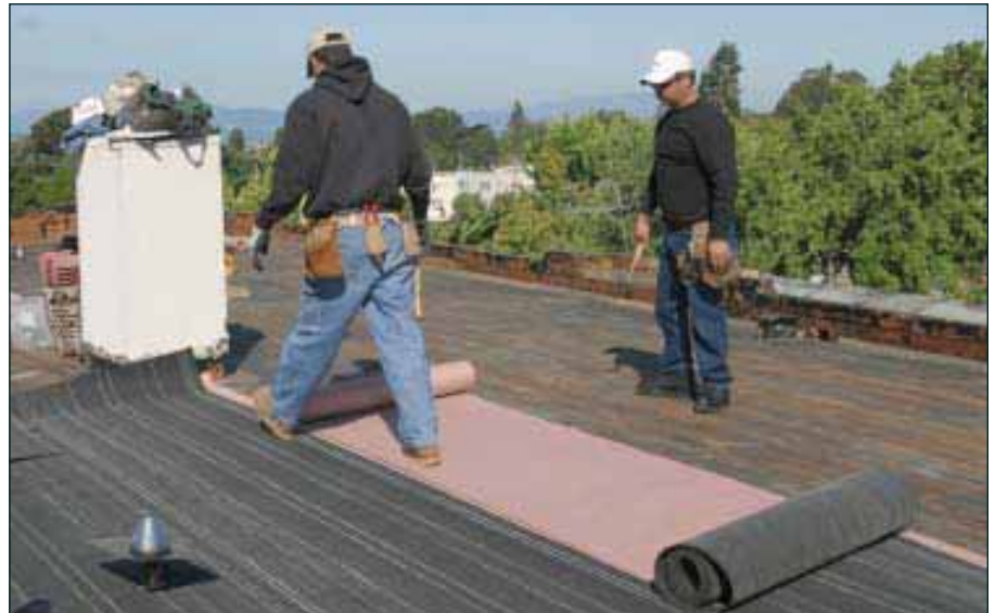
Figure 3. The base sheet goes over rosin paper and has 2-inch laps.
