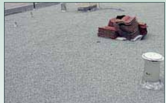
Figure 16. Here, one roofer lays down a thick flood coat of hot asphalt while another spreads crushed granite aggregate on top (left). Since the aggregate protects the roof from UV rays, no asphalt should be visible when the roof is done (above).
