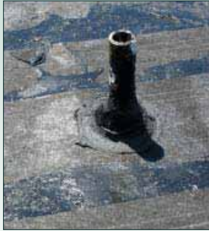
Figure 13. Most leaks happen at flashings and penetrations. To keep water from entering, crew members seal terminations with roofing cement (above). They then coat the cement with aluminum paint to protect it from UV rays (right).
