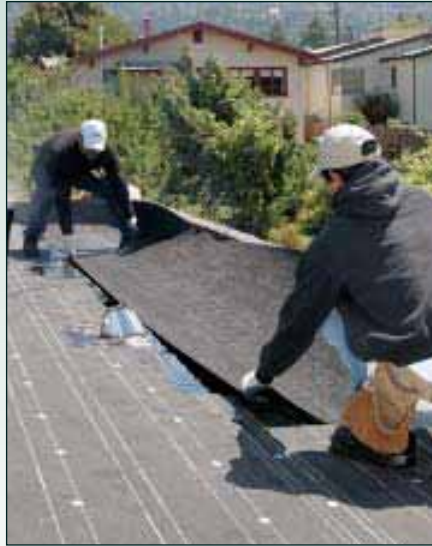
Figure 10. Hot asphalt is mopped onto the base sheet and felt in preparation for the next layer of material (left). These roofers are applying the first full-width piece of felt. There's already a 12-inch and a 24-inch strip below (right).
