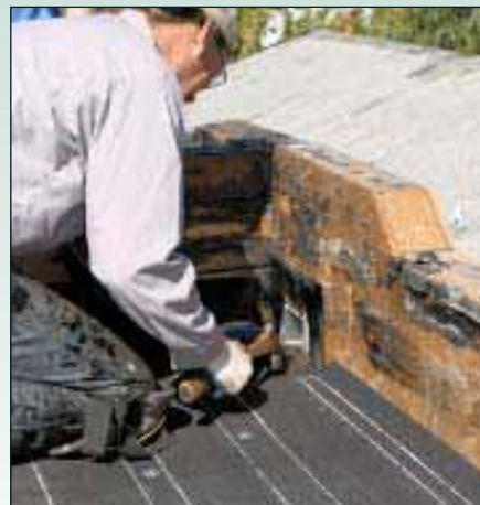
Figure 4. A roofer beds a scupper flashing in roofing cement (left) before fastening it over the base sheet (right).
