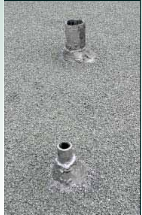
Figure 13. Most leaks happen at flashings and penetrations. To keep water from entering, crew members seal terminations with roofing cement (above). They then coat the cement with aluminum paint to protect it from UV rays (right).
