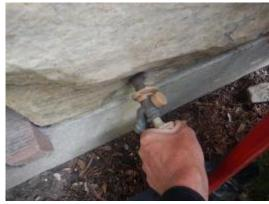
**RECOMMENDATION** - Secure the mounting flanges of the hose bib to prevent twisting.
