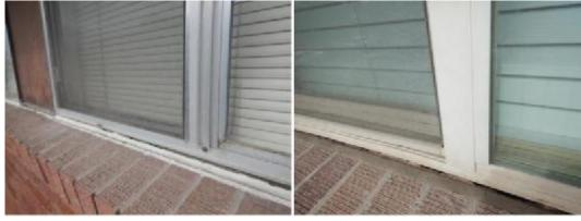
**RECOMMENDATION** - It would have been better if the windows did not terminate immediately on top of the brick so that an overlapping through the wall flashing could be used. But since it was done this way, then this caulking joint is critical. Obviously, the current joints have long been deferred. These must be touched up at least annually.
