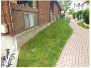
**GRADING** - **POOR** - Corrective action is needed. Currently, the east neighbor is NOT controlling the water on their lot and it flows down the slope directly into your foundation.
