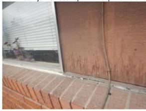
**FLASHING** -Look closely at the photo above and you can see that the through the wall flashing comes out about and inch and barely covers the brick.
