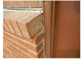
**RECOMMENDATION** - The door frame to brick and siding joints need to be recaulked.
