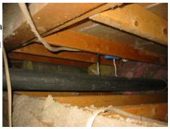
Type: Blown-in Cellulose. Total Thickness: 4"-6". **ATTIC INSULATION:**
