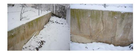
There is a west lot retaining wall installed. There is a vertical crack but only a little
