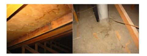
There is past leakage at the vent pipes, flue and swamp cooler. Monitor these for any
