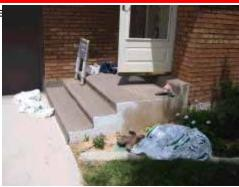
**HANDRAIL:** There is no handrail installed = Consider adding for safety.
