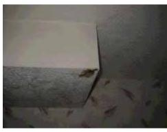
**FLOORING:** The flooring is damaged and discolored from a longe term toilet base leak.
