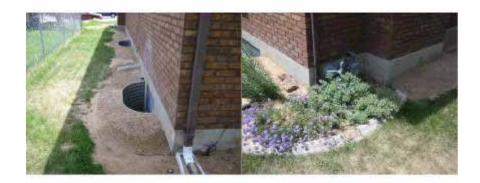
The perimeter grading has just recently been corrected. They have installed a sandy soil around the majority of the foundation. The SE corner still needs corrective action since a downspout discharges into the planter bed and water is trapped near the foundation. The grading should be corrected and a downspout needs to be extended with a drain line.
