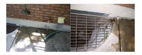
The window well set into the rear patio needs to be re-excavated. The typical installation of the window wells includes the removal of 14-18" of earth below the window sill and then filling the well with gravel. This allows water to collect and soak in to the earth without over filling and flooding the basement.
