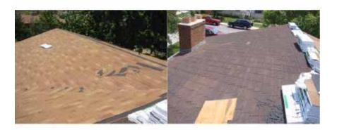
The roof is two thirds complete. The exposed older roof was really deteriorated. The only thing missing with this new installation is increased attic ventilation. The attic was very hot today and you should consider upgrading the attic ventilation. This is usually accomplished with either ridge or roof mounted static vents.
