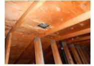
FIREWALL: There is one communal type attic, instead of the modern recommended divided and firewall protected attics. The drawback is that if a fire breaks out and gets
