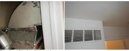
There is no filter installed on this system.
