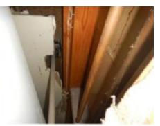
Yes = Did Not Test. They routed the discharge into a drain pipe inside the wall cavity.
