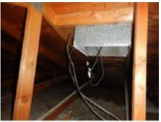
They aborted the ducts. You can see prior staining and the aborted electrical wiring that is still live.
