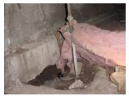
WATER MAIN TYPE & SIZE: The portion viewed was Galvanized. The exposed main line was 3/4" diameter
