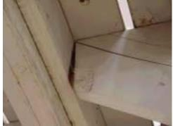
RISER/TREAD RATIO: Good. The lower block stairs are too steep and they have no handrail installed =
